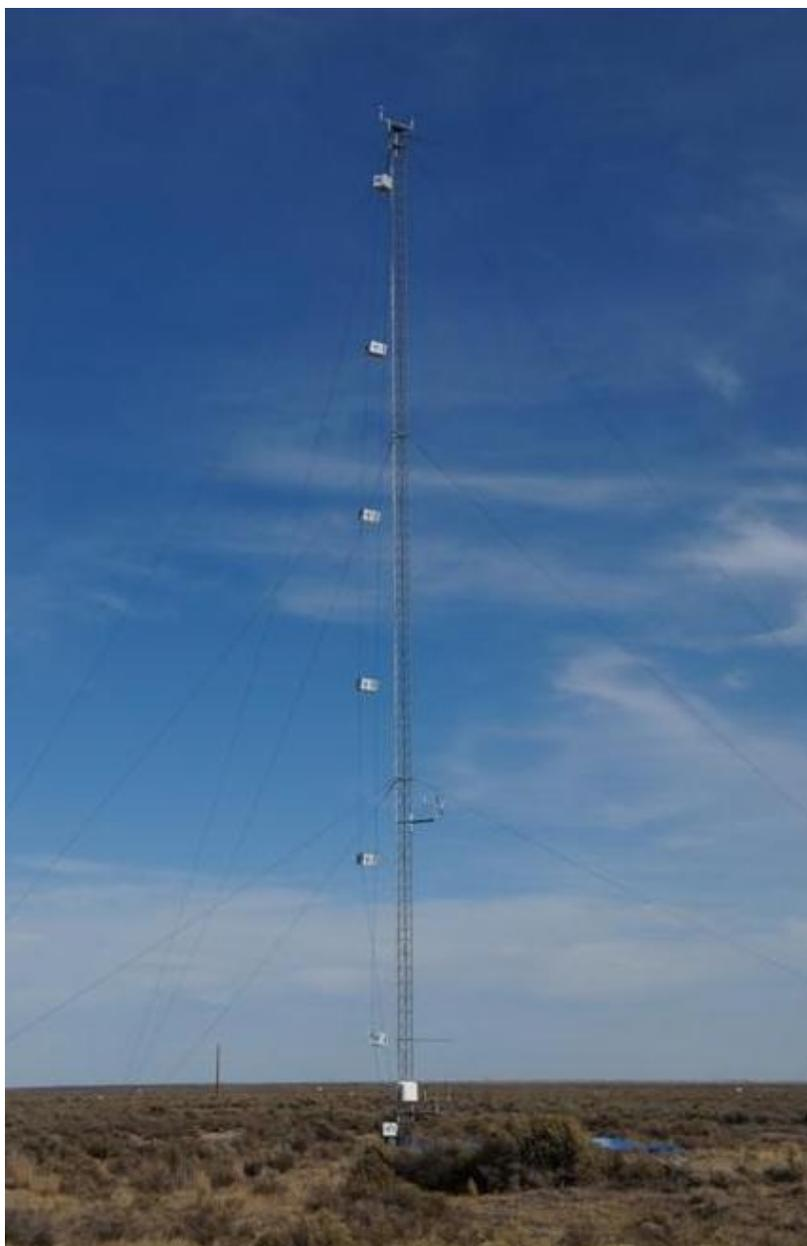
Figure 53. 30 m command center meteorological tower (COC).
