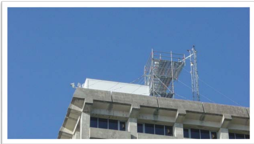
Measurement scaffold atop the Moody Tower on the University of Houston campus.
