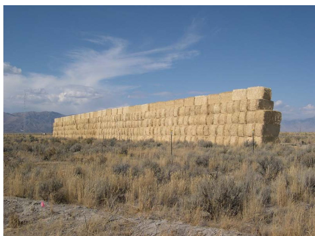
Figure 3. Mock sound barrier was constructed of 300 1-ton straw bales 6m high by 90m wide.
