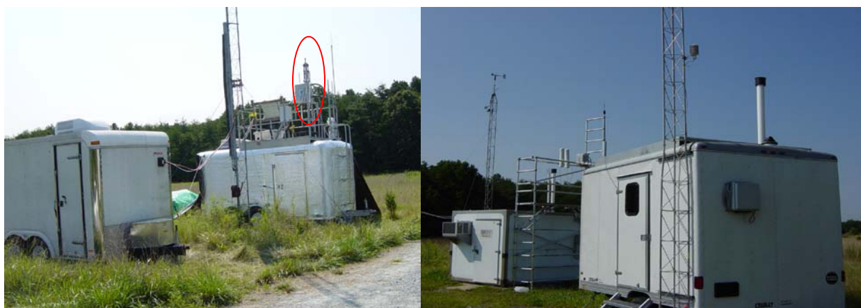
Fig. 4. Instrument shelters at the Beltsville sampling site. ADS are shown (red circle) attached to roof scaffolding in the first image.
